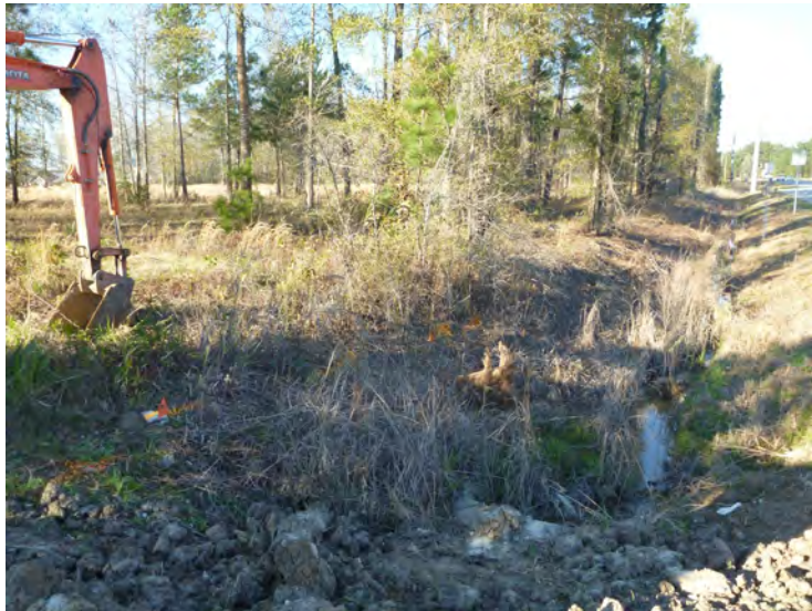
Photograph 3. Wetland 2, facing north, northwest of intersection of SR 21/Augusta Rd and Rice Mill Rd.
