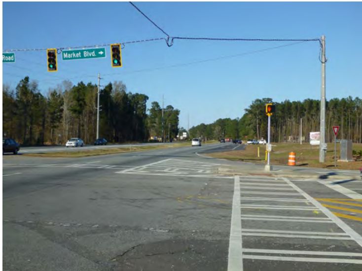
Photograph 11. Intersection of SR 21/Augusta Rd with Rice Mill Rd and CS 705/Parkside Boulevard.
